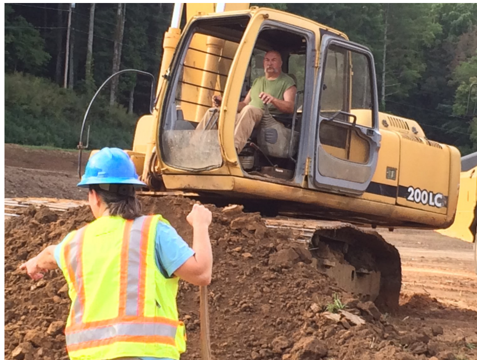
Gary Scott, Owner of Appalachian Construction working with a Geologist at Parker Meadows Recreation Complex.
